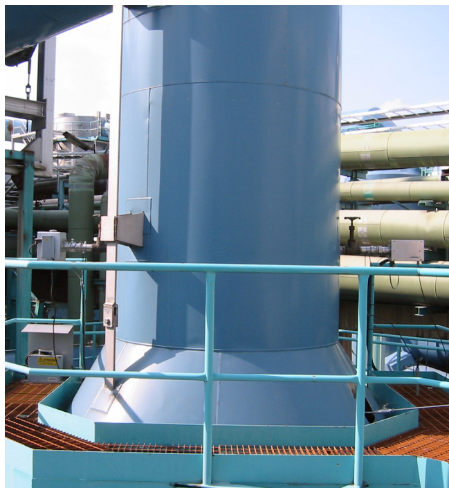
A cross-stack installation, showing the emitter and receiver
